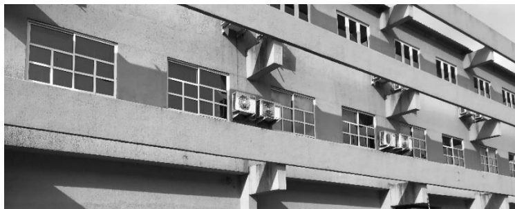
Figure 7.2.1. Case study building A
