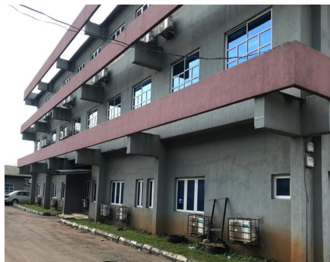
Figure 2.6B Typical office building with 21 air conditioning units on one facade (captured by the researcher)
