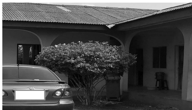
Figure 7.2.2. Case study building B
