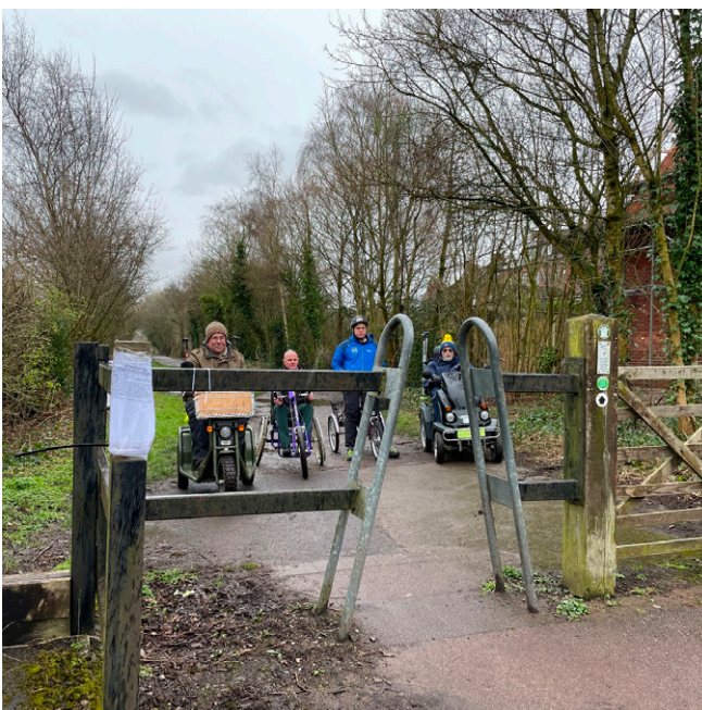
Figure 19 A group on mobility scooters faced with access barriers at Whitbarrow Road, Lymm
