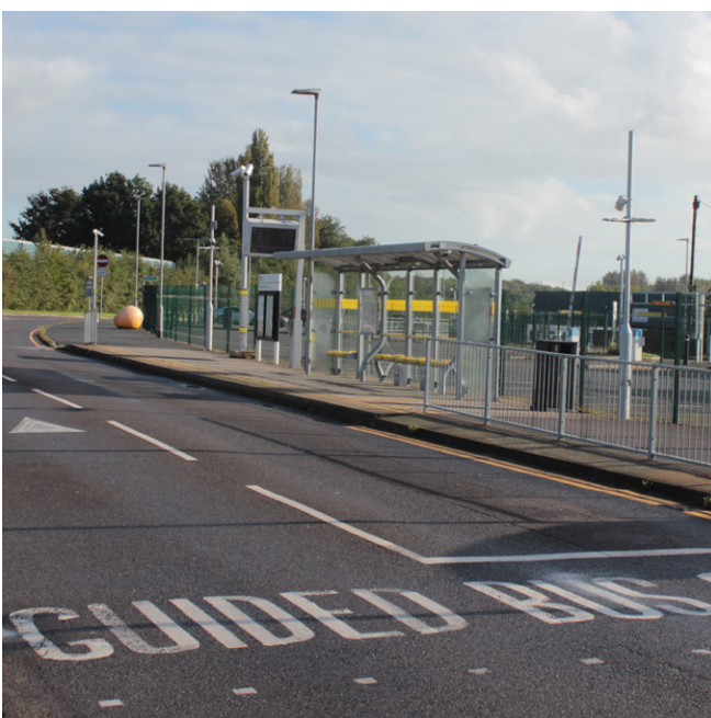
Figure 16 Start of the guided busway at Bond Street
